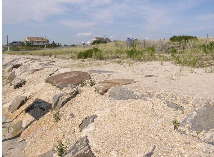
Portion of Cape May Seawall in Area 1.
