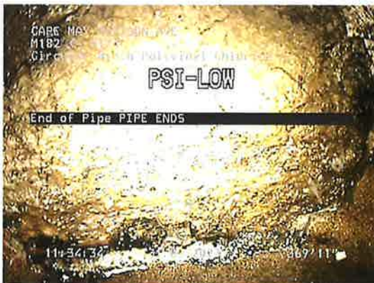
M182_M174_3312023 120938 PM_AEP_60.jpg, 00:21:37, 369.92ft End of Pipe
